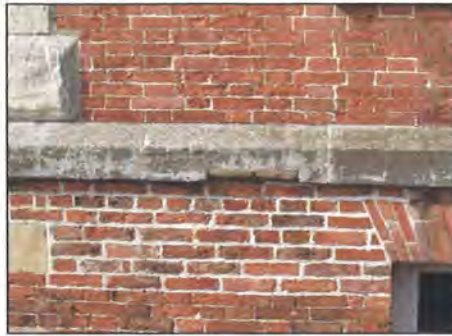
Plate 15: Example of a Repair Where the Original Bricks have been Reused
