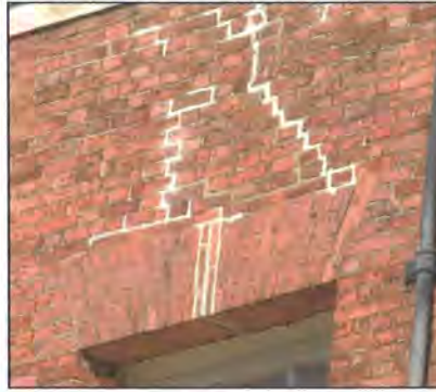
Plate 7: Example of Brickwork Lintel that was Repaired Using the Original Bricks
