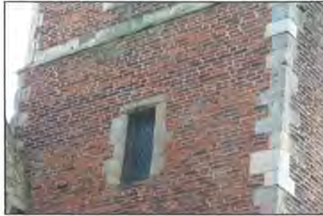
Plate 5: Example of Recently Repointed Brickwork
