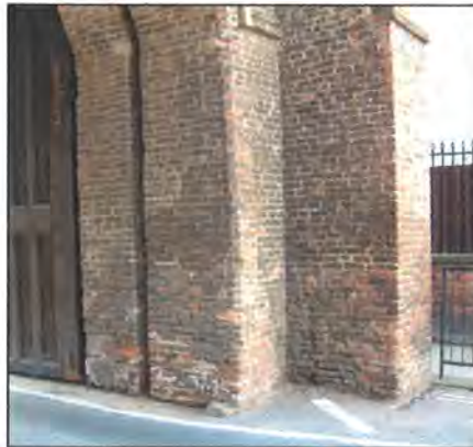
Plate 4: The Brickwork at North Bar
