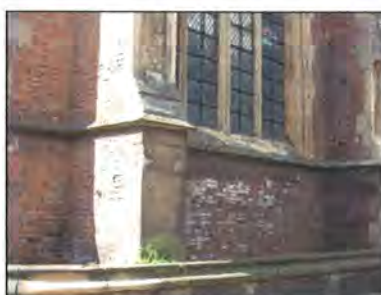
Plate 2: The North Side of the Chancel at Holy Trinity Church
