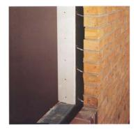
Heads, cills and reveals required allowance for projected movement too, and at the heads of window in storeys five and six, bed joint reinforced brick lintels have been used. For spans of up to about 2.1m these are easy to design and construct and give complete independence between brickwork and timber-frame at the upper storeys.
