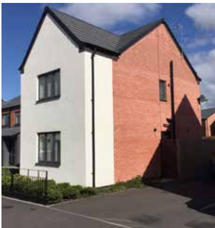
Concrete Brick - Note the joint on the gable.
