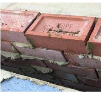
**Tipping and Tailing Brickwork**
