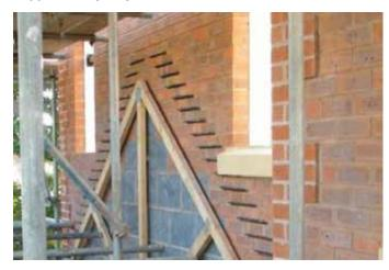
Flat Roof Flashing Tied in to Cavity Tray
