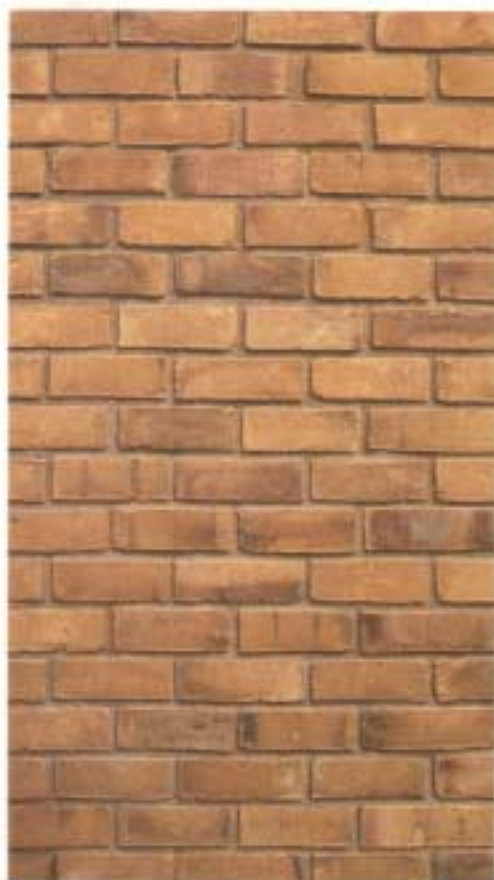
Brickwork with recessed joints
